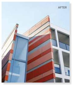
This five storey modular wall would be a bland monolith without the depth and colour of Aerostone cladding. Manufactured from Hebel, the cladding was supplied as 25mm thick panels in modular sizes. Using a combination of applied cladding and on-site routing, the face of the building was transformed with stepped and negative lines. Acrylic texture coating was applied in three colours to create a seamless finish. The result was a visually impactful, three dimensional effect.
